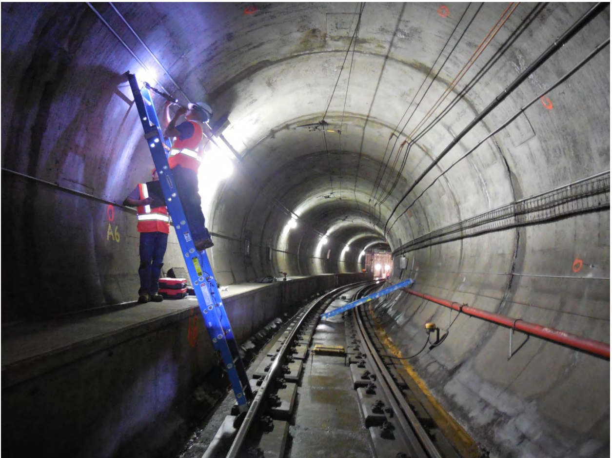
Figure 7-51 : Tunnel Mayfair - Edmonton LRT
