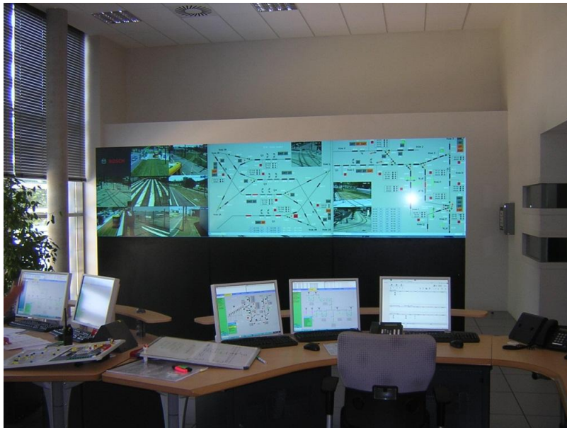
Figure 4 PCC du tramway de Mulhouse – France
