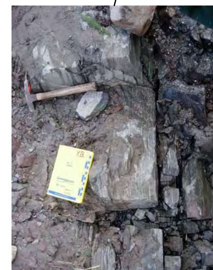
3 OPEN JOINTS, CALCITE FILLED SPACING : 0.05 TO 0.5m GREENISH MASSIVE BEDS OF MUDSTONE
