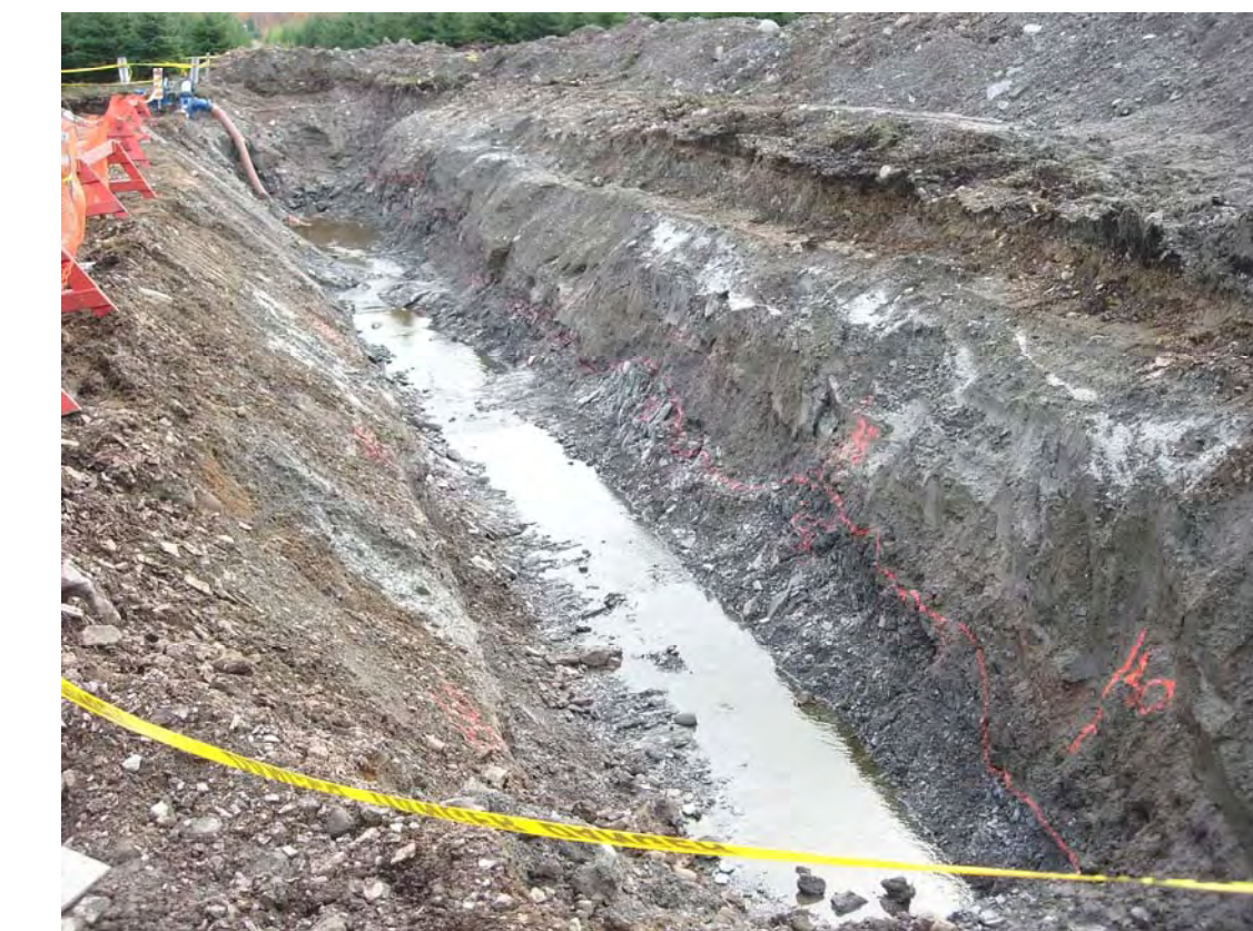
VIEW OF TRIAL EXCAVATION TR-B-05 LOOKING SOUTH
