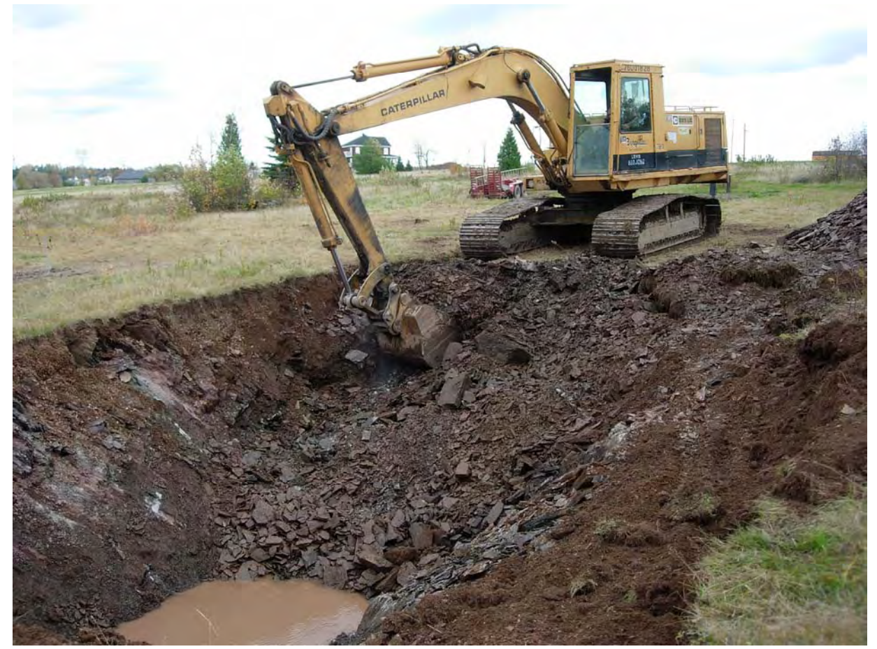
VIEW OF TRIAL EXCAVATION TE-A-05 (LOOKING SOUTH-EAST, DURING EXCAVATION)
