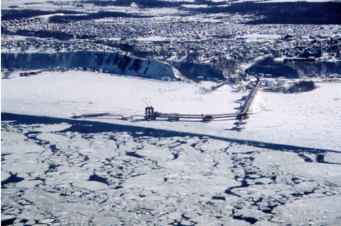
Figure 11.1 Aerial picture of Ultramar wharf taken on March 6, 2003
