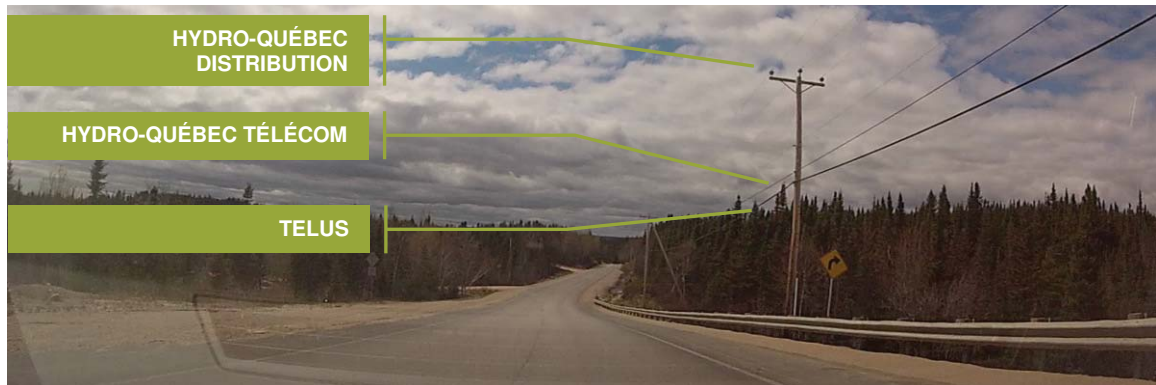
Figure 15 Poteaux de distribution (route 389, km 17)
