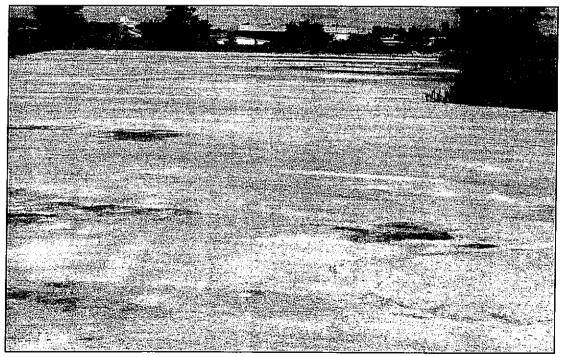
The Posi-Shell® Cover System can be effectively used as a barrier to dramatically reduce airborne emissions from volatile organic compounds, aldehydes, ketones and alcohols from exposed waste surfaces. Posi-Shell forms a resilient surface after curing and can reduce the chemical emissions of these compounds by as much as 97%.
