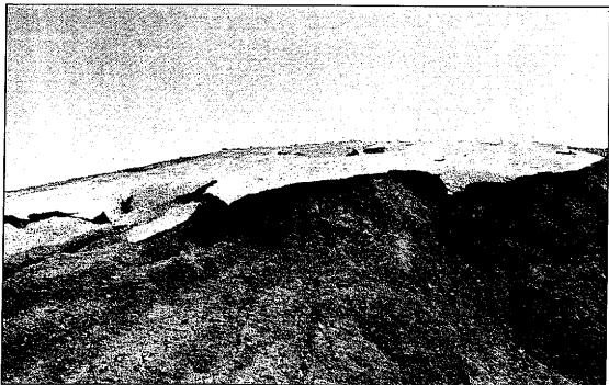
Posi-Shell® Cover has been effectively utilized to protect outdoor coal piles from water infiltration and to eliminate windblown dust from the piles. Economic benefits include increased BTU value and elimination of complaints and costs related to cleanup of offsite coal dust.
