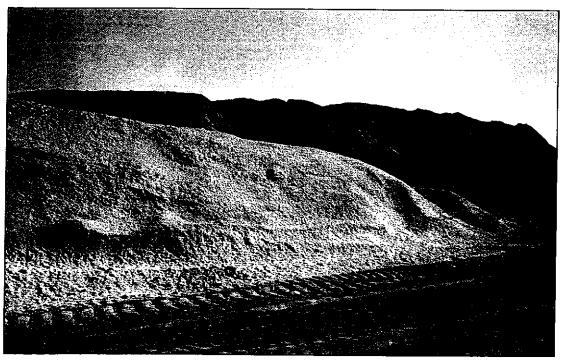
Posi-Shell® Cover has been successfully employed at numerous federal Superfund sites to reduce or eliminate emission of volatiles from excavations and material piles. The Posi-Shell® covering has also been employed at these sites to provide erosion control and to eliminate wind-borne dust transfer of contaminated materials.
