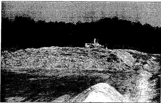
Posi-Shell® provides an extremely effective means of coating the exterior surfaces of compost piles during the active composting period. The lime content of the Posi-Shell® mixture aids in the reduction of odors and the Posi-Shell® coating eliminates windblown debris without interfering with the biostabilization processes.
