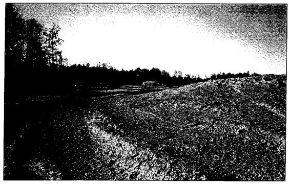
Posi-Shell® Cover provides a hard-shell coating to effectively protect against wind and water erosion. Typical applications are on intermediate and preclosure areas of landfills and other large sloping soil surfaces.
