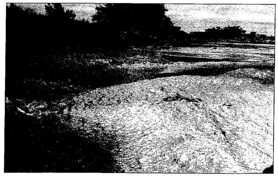
Posi-Shell® Cover is uniquely suited to coat sludge or tar lagoons which require application from the outside perimeter of the lagoon. This procedure controls the emission of volatiles, thus reducing odor while eliminating rainwater runoff contamination.
