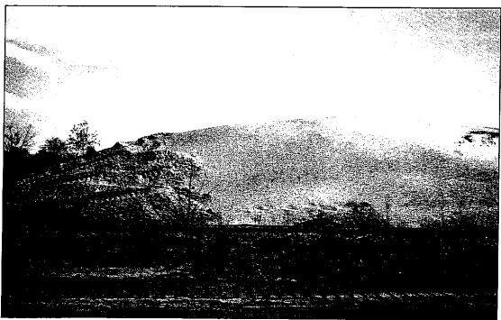
Posi-Shell® Cover is very effective in the prevention of dust migration and water erosion from outdoor contaminated soil piles. The cementitious coating protects these piles from high winds and rainwater infiltration, thus eliminating the cost of subsequent remediation activities.
