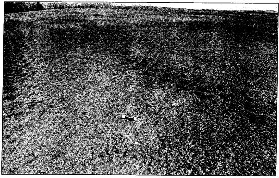
Cementitious Posi-Shell® spray-on cover eliminates the need to physically traverse wet or unstable piles of ash material. An effective long term cover that can be quickly and easily placed over these materials while eliminating the operational difficulties and high-volume consumption related to soil covers.
