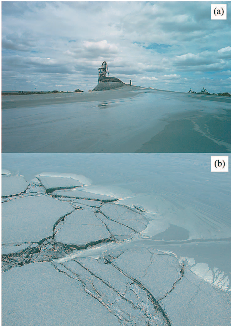
Fig. 6. Pictures of paste tailings: (a) end-pipe discharge from one of the towers, (b) new layer of paste flowing over a desiccated sheet of paste.
