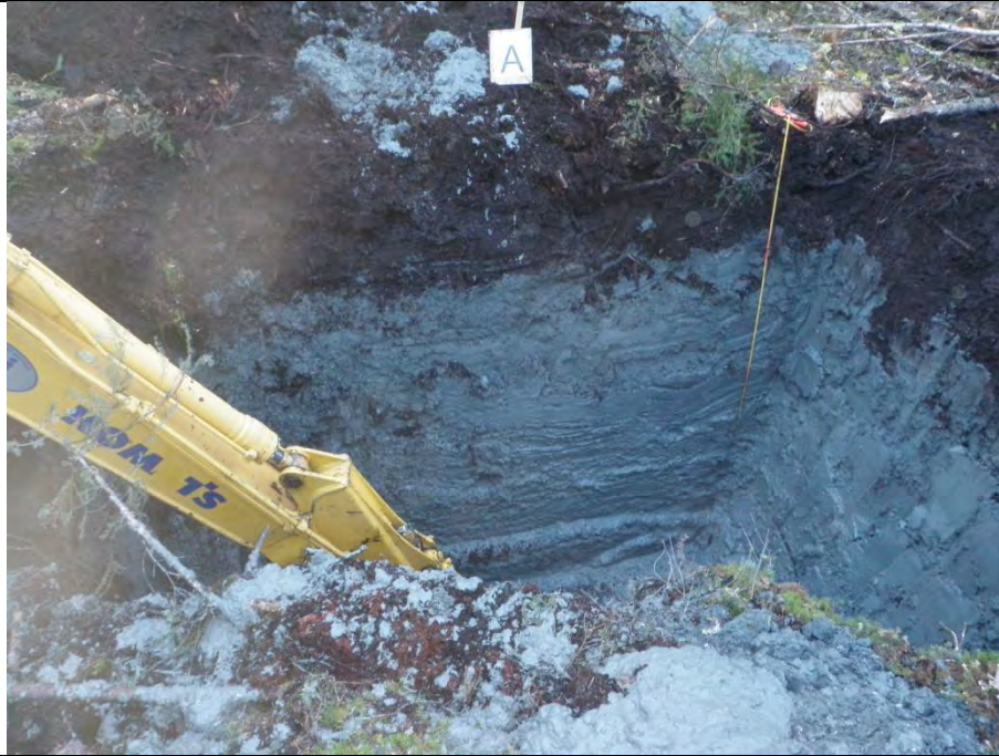
Side A : North Wall
