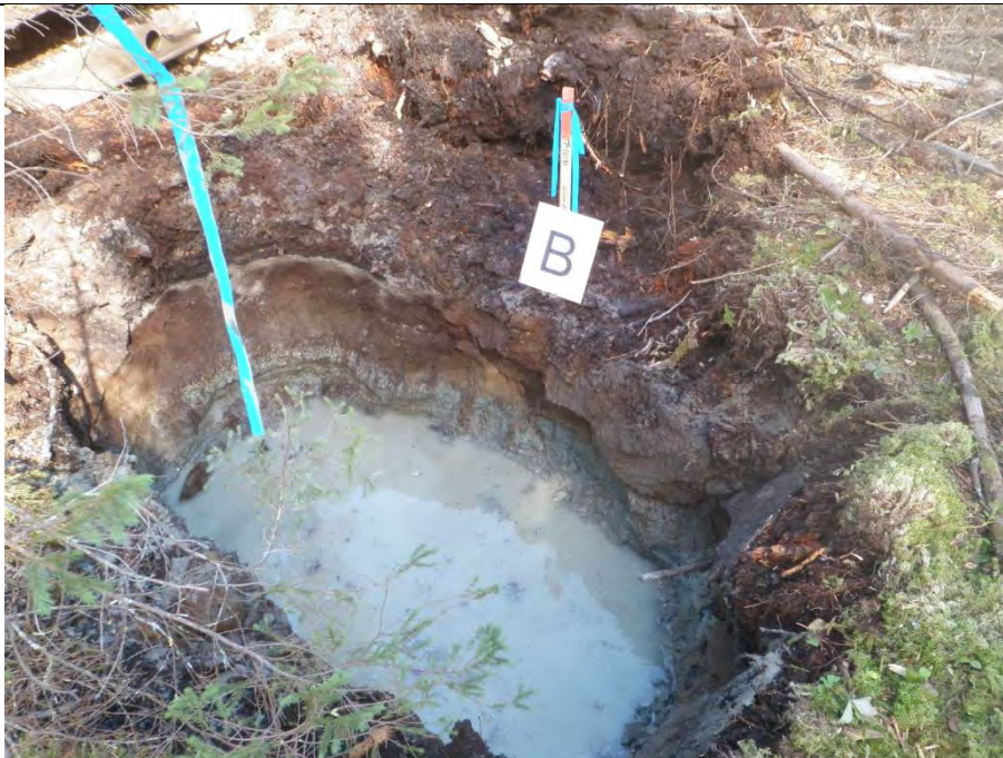
Side B : North-East Wall
