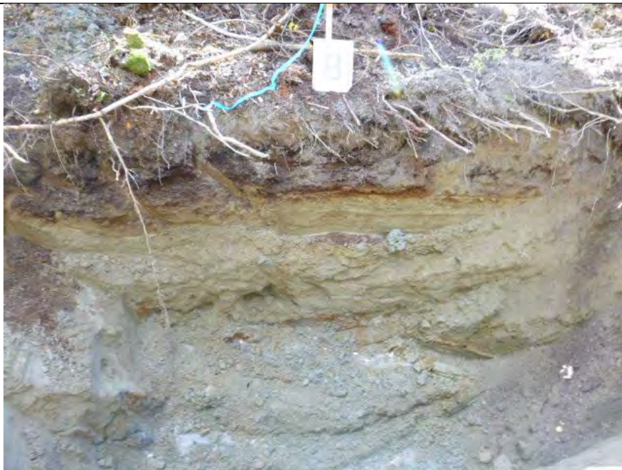
Side B : South-West Wall
