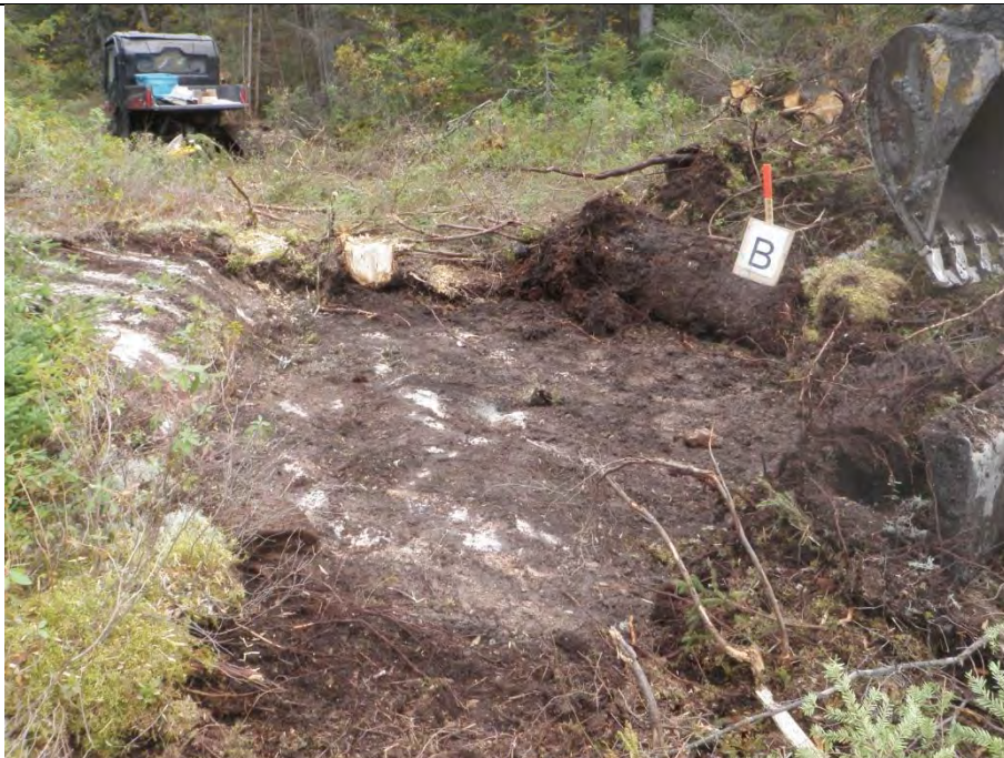
Side B : South-West Wall
