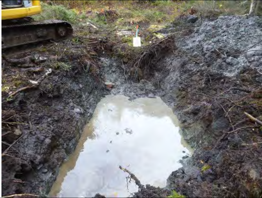
Side A : North Wall
