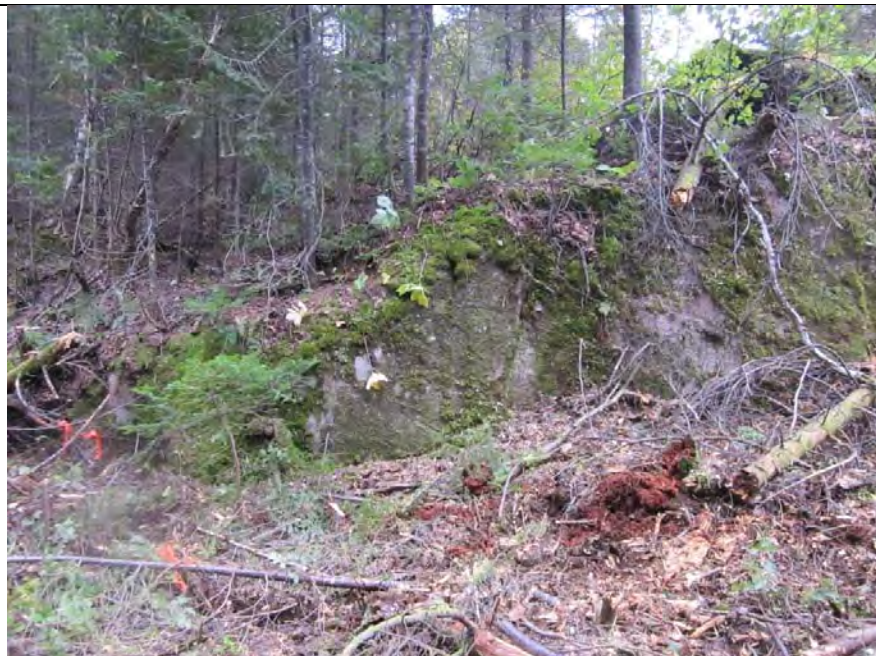
OB4_P04: View in the North direction. Between GPS no. 42 and 43, abrupt rock walls between 0.9 to 3.6 m high. Small fragments are detached from the outcrop.
