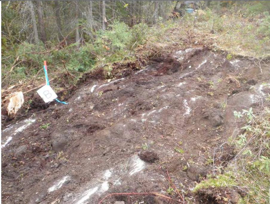
Side B : South-West Wall
