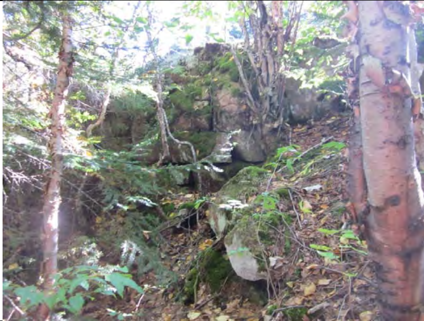
OB7_P03: View in the South direction. Rock wall from 4 to 5 metres high. Some fragments detached from the rock wall.
