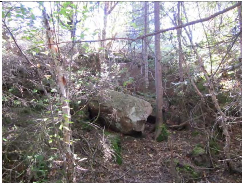
OB7_P04: View in the South direction. Rock wall from 4 to 5 metres high. Some fragments detached from the rock wall.
