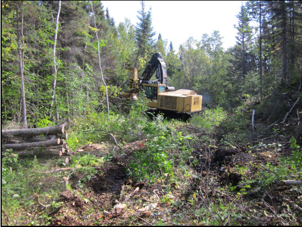
Figure 2 - General view of the land-clearing work
