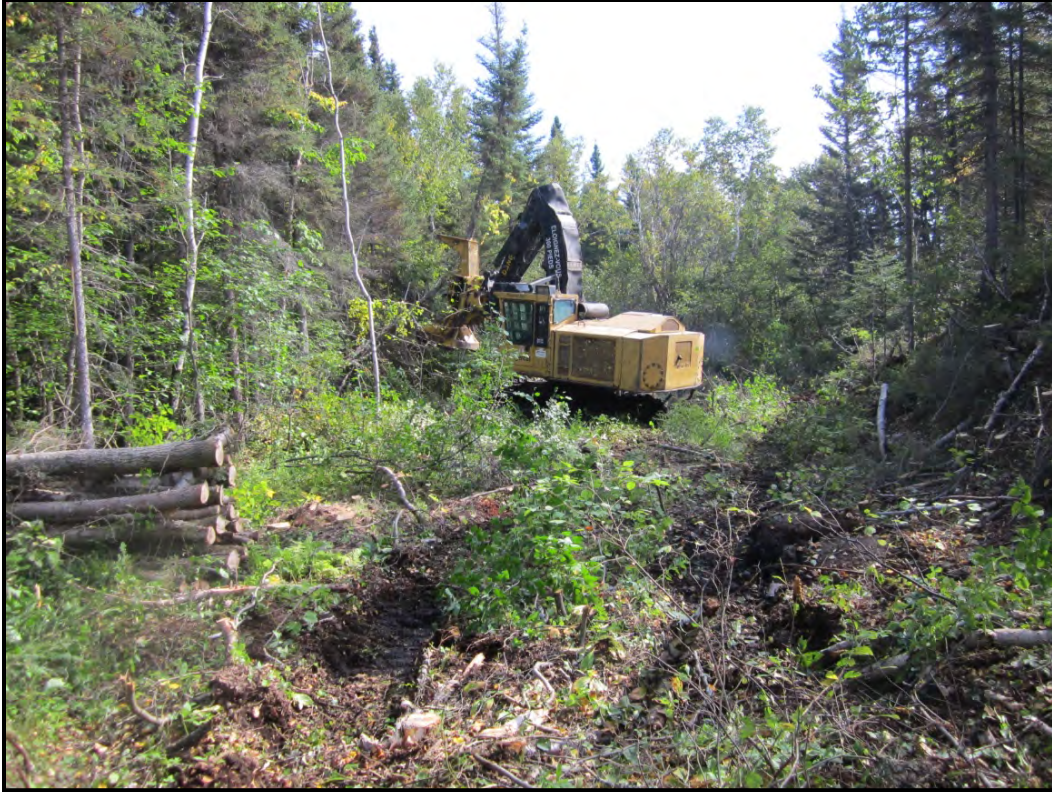
Figure 2 - General view of the wood-clearing work
