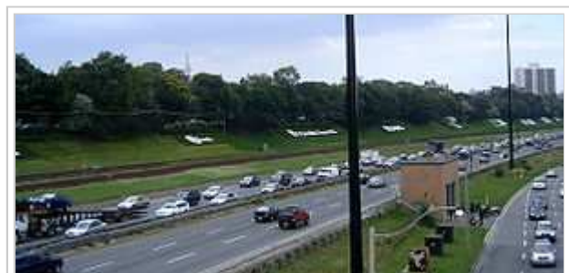
View of the Expressway, west of downtown Toronto, from the pedestrian overpass at the foot of
