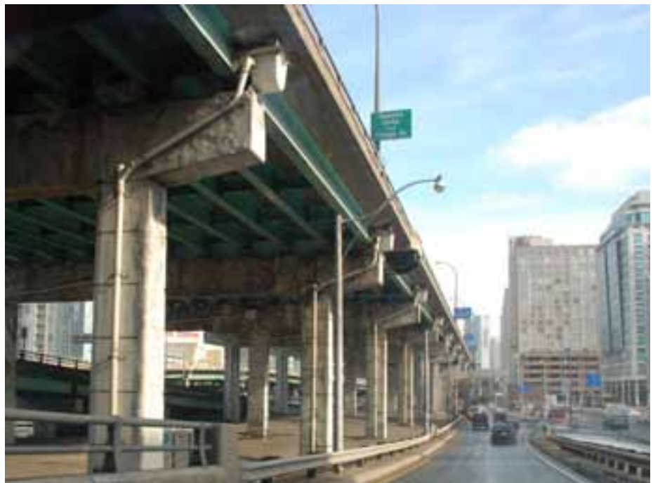
Gardiner Expressway in downtown Toronto.
