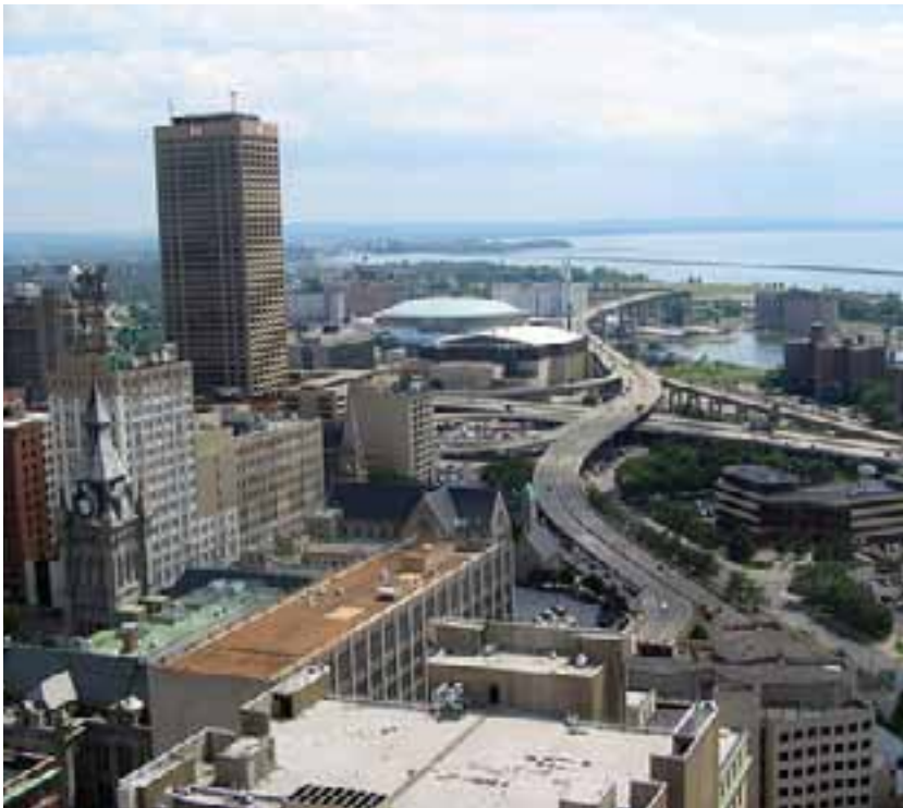
View of Skyway facing south.
